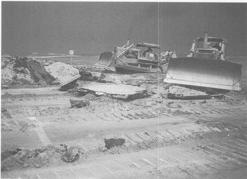
Contractors repair roads in Kuwait.
