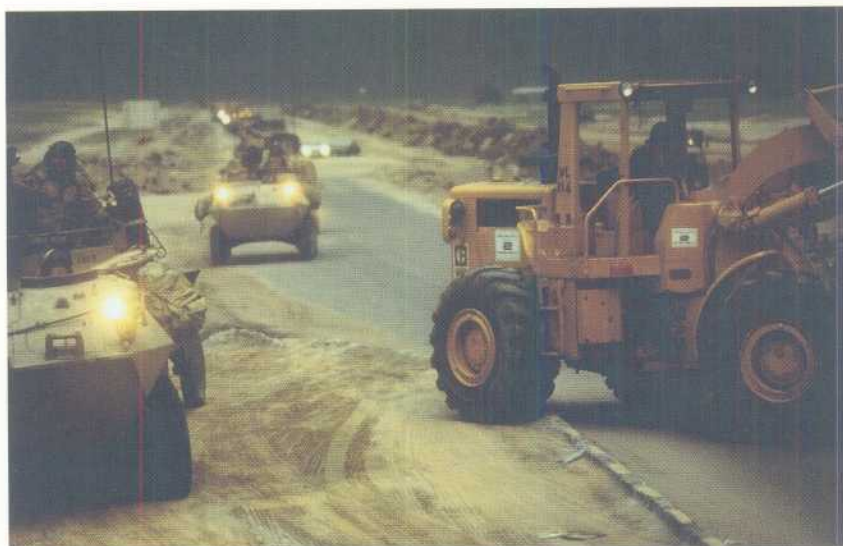
Power cable repair south of Kuwait City
