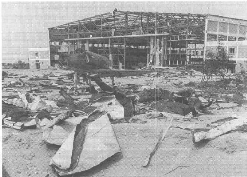
A destroyed aircraft hangar at Al-Jaber Air Base
