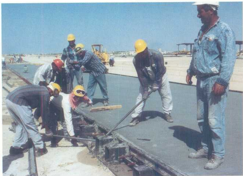
Repair work at Al-Jaber Air Base
