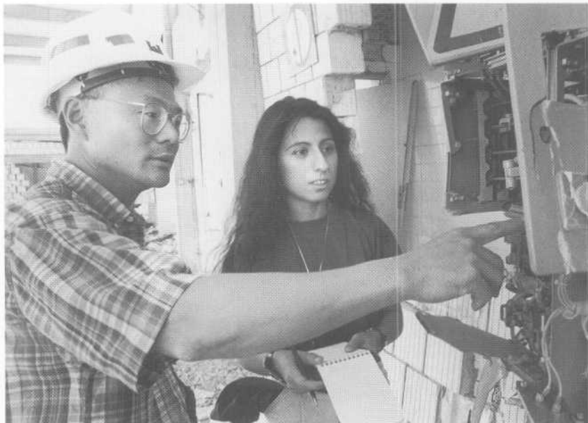
Jim Wong, U.S. Army Corps of Engineers, and Suhalla Marafi, a Kuwaiti engineer, inspect electrical damage at Ali Al-Salem.
