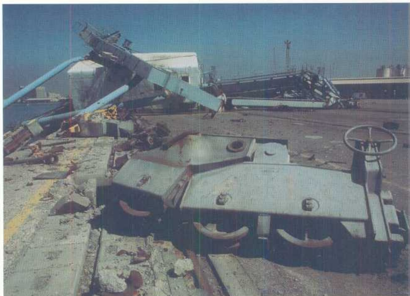
Facilities at Shuwaikh port were badly damaged.
